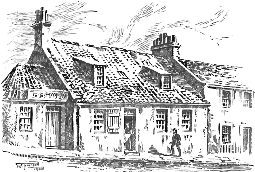
House where Web-beaming Machine was first started, 1840 : also birthplace of Dr. A. Carnegie, Moodie Street.
