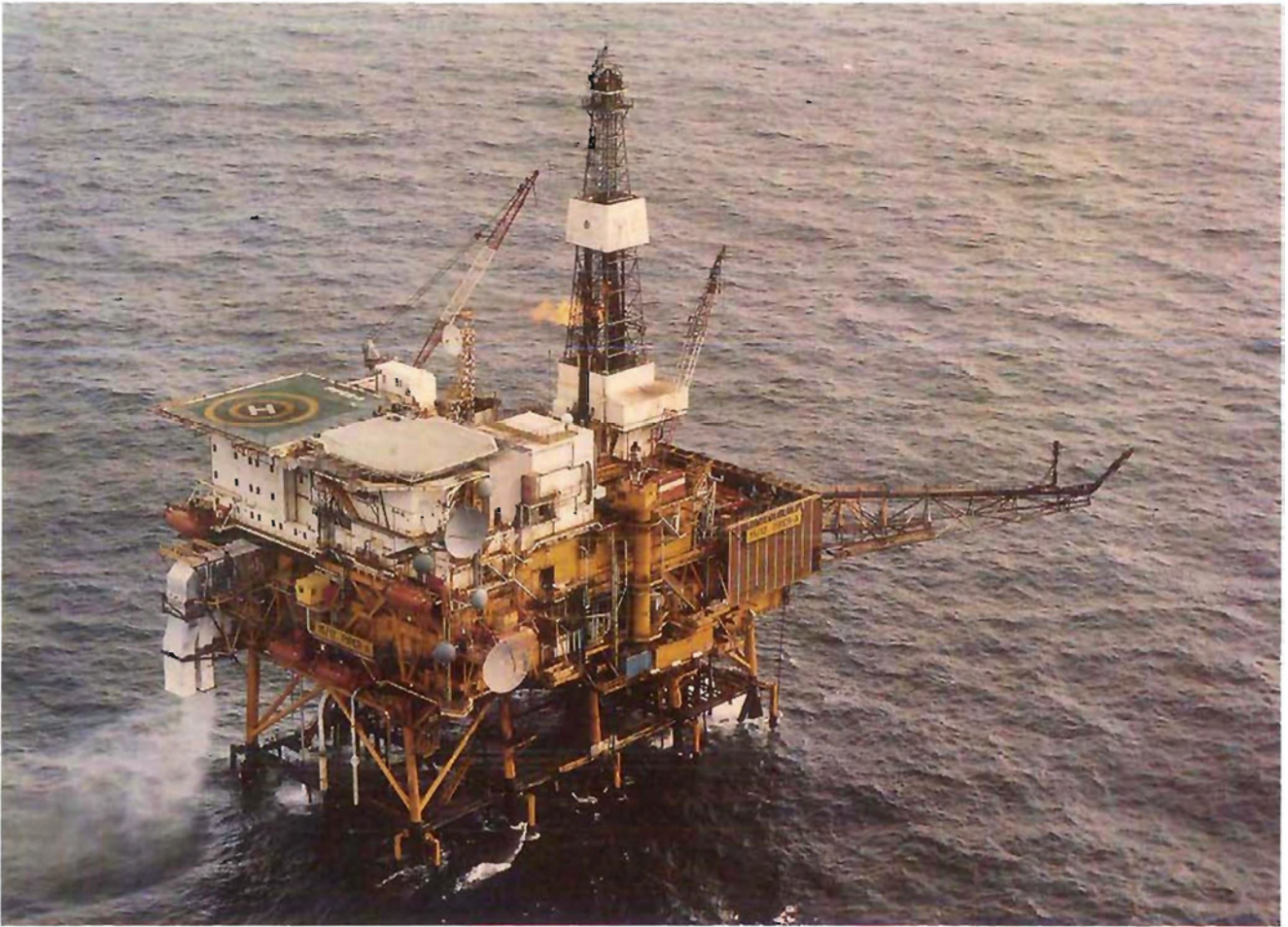
Plate 3 The Piper Alpha platform: view from the north-west.
