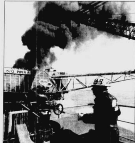
Fred Adair aboard the Tharos; his task is blocked by tons of debris.
